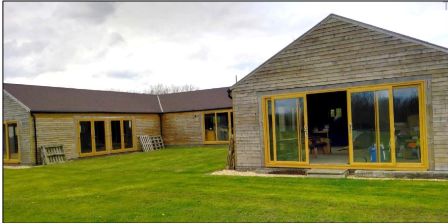
Building as noted during enforcement investigation (complete with glazed windows and doors as opposed to roller shutters).
